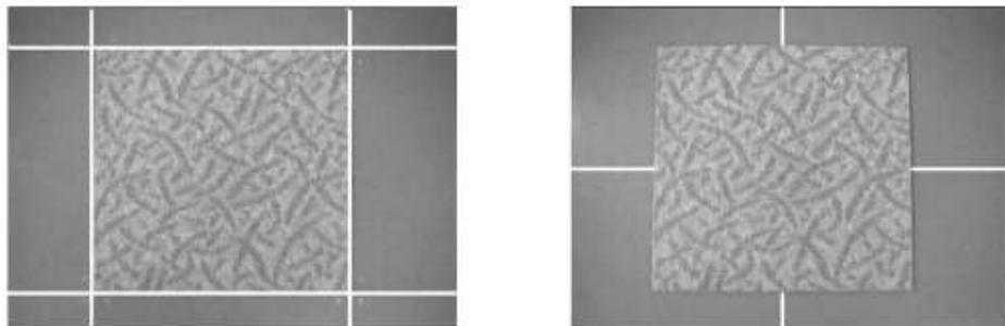
Figure 19 - Two different modes of carpet tile installation on raised floor panels: aligned (left) and offset (right). White lines indicate the floor panel edges.
